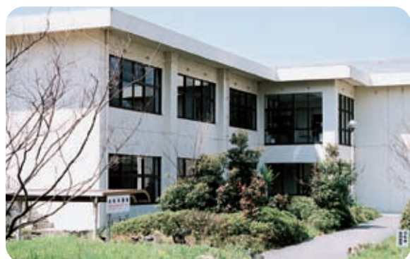
共通講義棟 School Building (F Zone)
