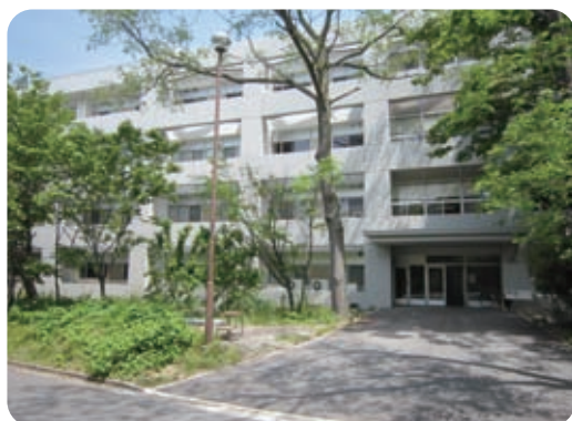
1号館（A棟） School Building No.1 (Azone)
